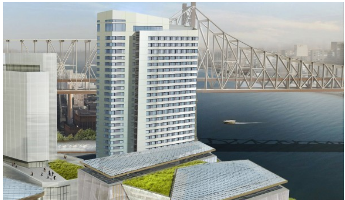
A rendering of Cornell University's Tech Campus on Roosevelt Island in NYC, which will be the world's first Passive House high-rise. It will open in 2017. xxiv
